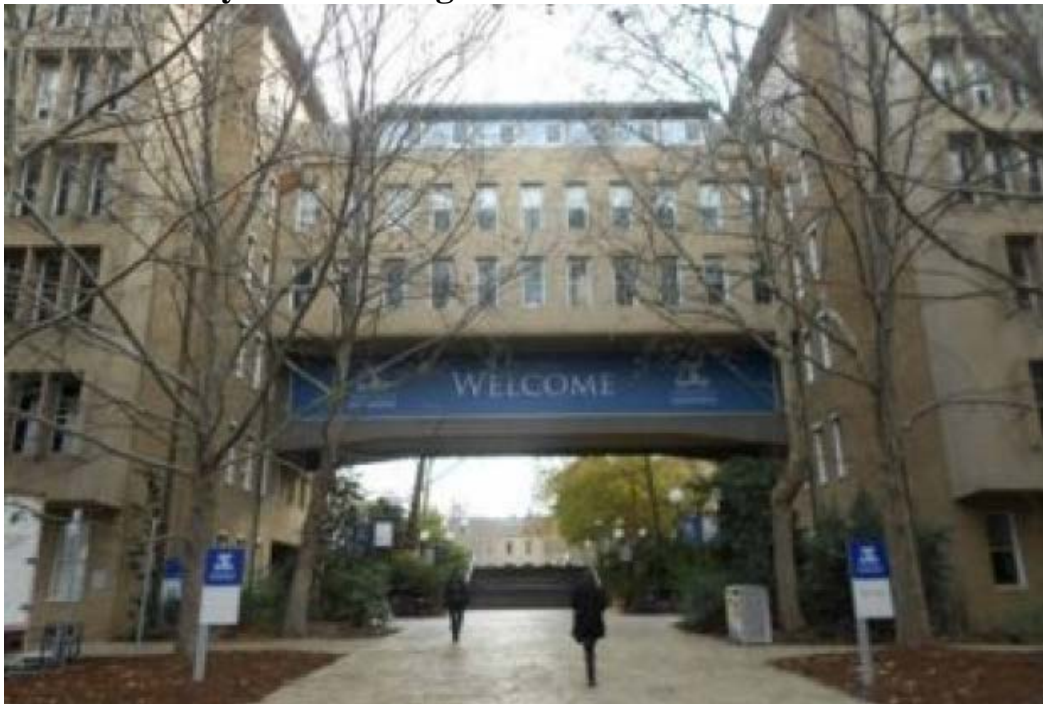
The Medley Building Photo: Lostoncampus.com.au
